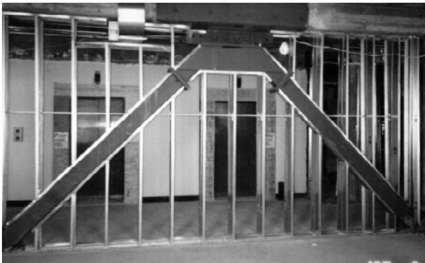
Figure 5: Pall friction-damper at top of chevron brace
