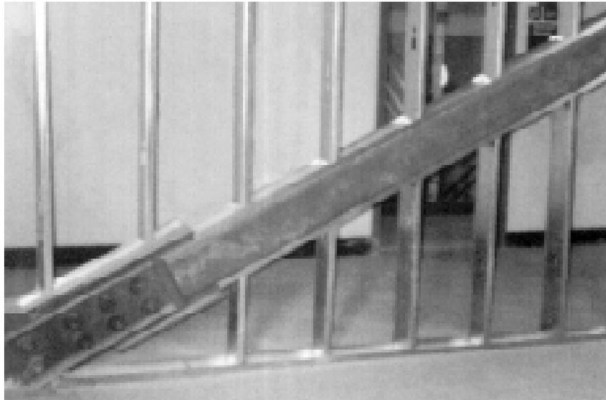
Figure 4: Pall friction-damper at bottom of single diagonal brace
