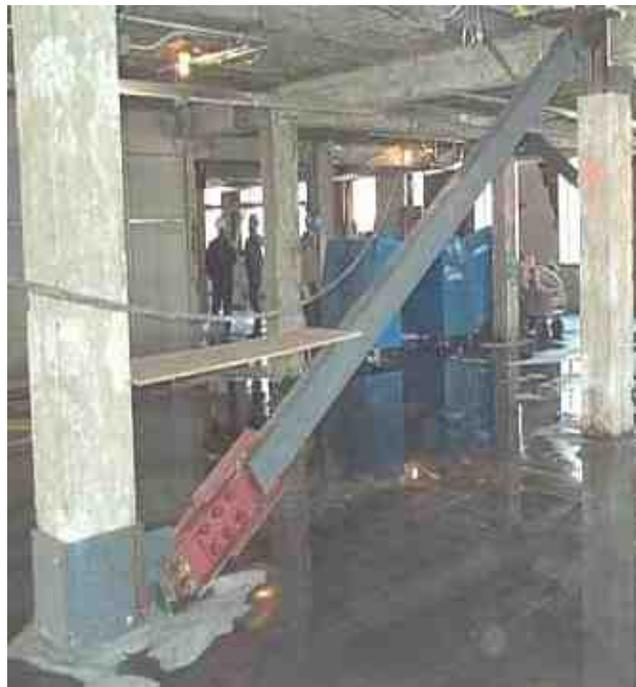
Figure 4. Friction damper at bottom of single diagonal brace
