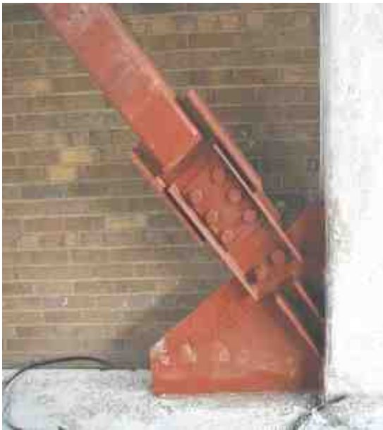
Friction damper in single diagonal bracing
