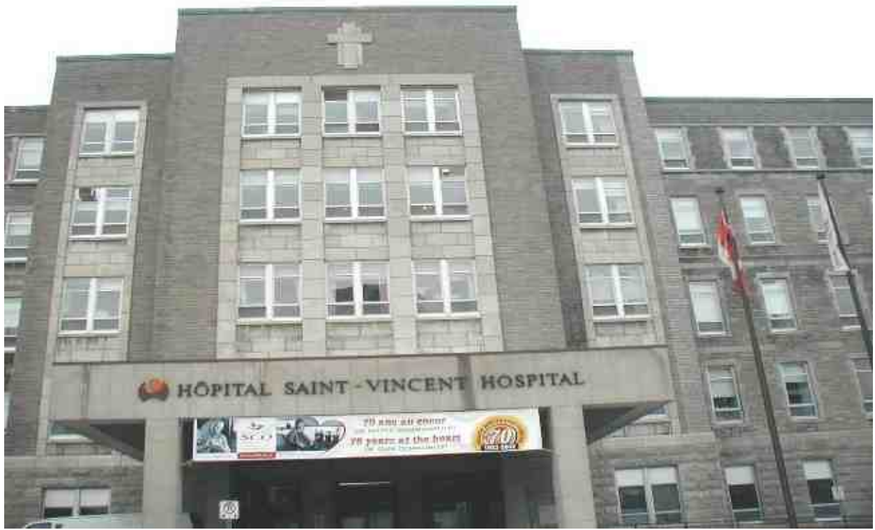
Figure 1, Front View of Wing-B (Partial)
