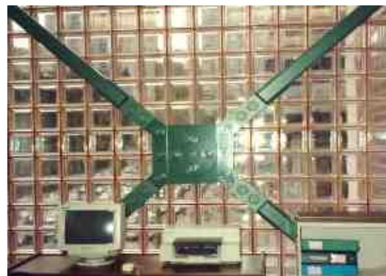
**(b). Pall Friction Damper in Cross Bracing**
