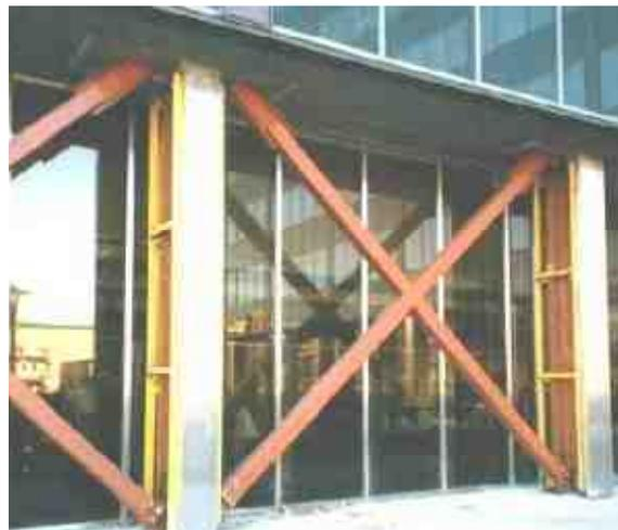
**(b). Pall Friction Dampers in Bracing**
