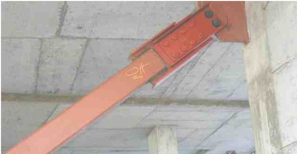
Figure 4. Typical Pall Friction Damper in a single diagonal brace.
