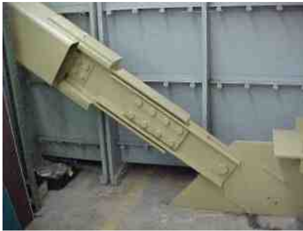
Figure 8. In-line Pall Friction Damper
