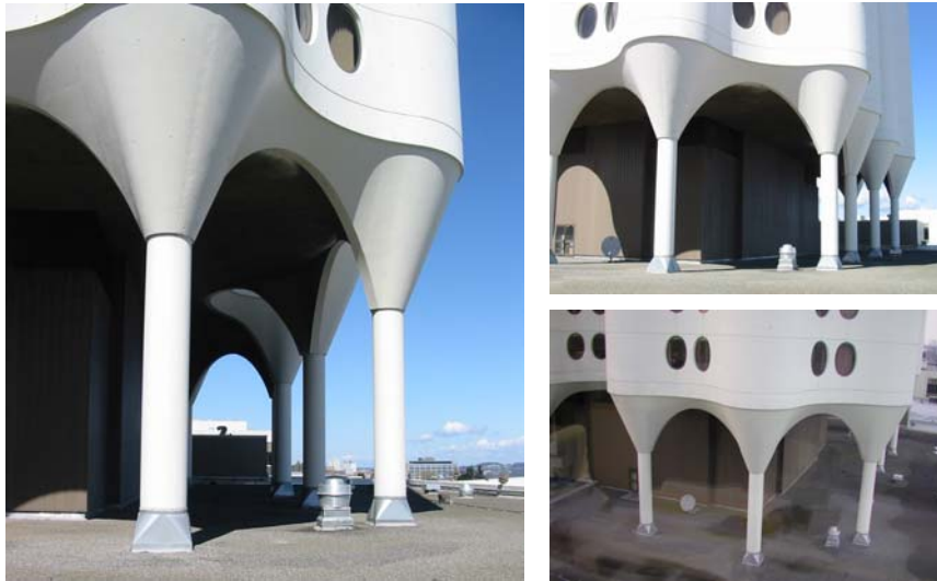
Figure-3. Existing Building Soft-Story
