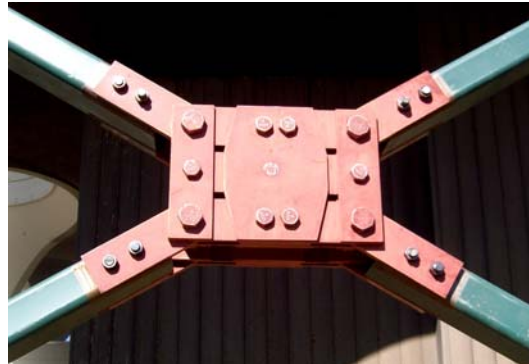
Friction Dampers Installed
