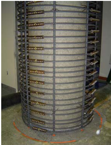
Figure-9. Concrete Column Enlargement Before and After
