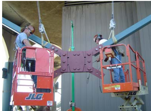
Figure-10. Steel Jacket and Damper Installation
