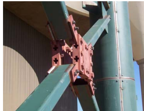
Figure-10. Steel Jacket and Damper Installation
