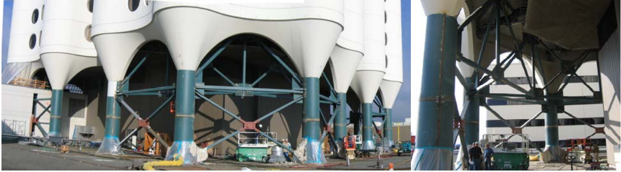
Figure-11. Completed Damper Installation
